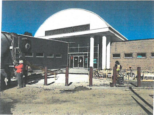
South Entrance Step Removal
