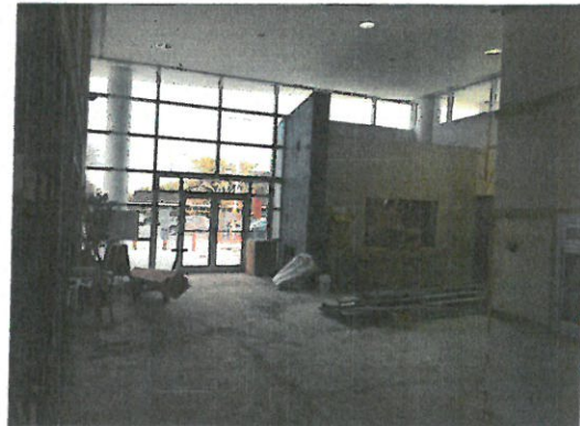
Lobby Work Area
