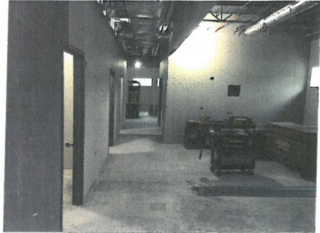
Interior Office Wall and Duct Work
